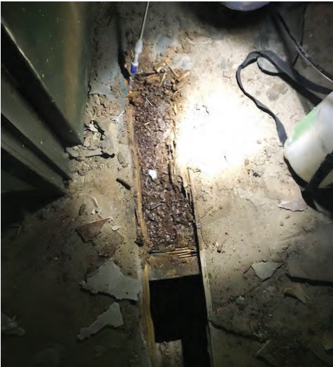
A termite infestation in the Waikerie Institute's former projector room. PHOTO: supplied
