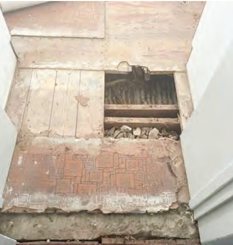
Termites have damaged the kitchen floor in the Waikerie Institute making the area unsafe for the Santa's Cave Shop this year. PHOTO: supplied
