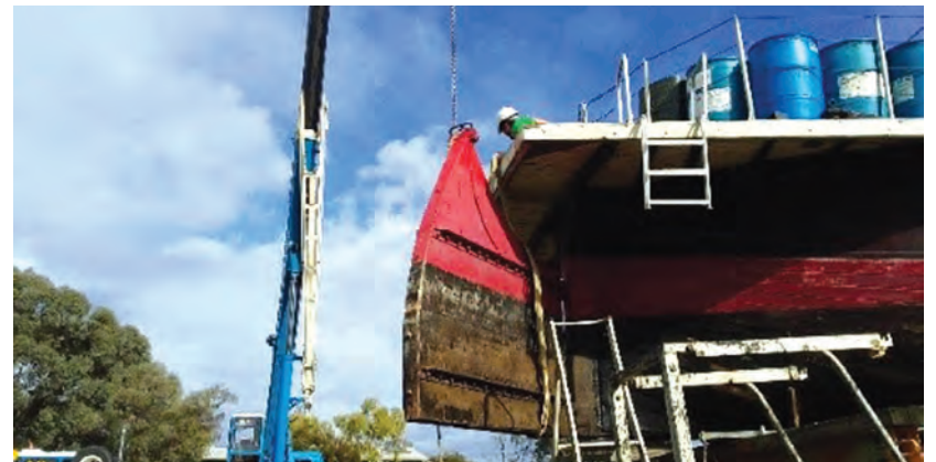
An unscheduled major overhaul of the rudder was completed while the PS Industry was on the SA Water slipway in Berri. PHOTOS: supplied
