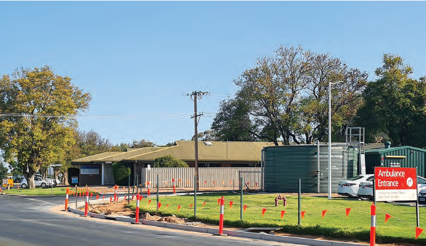
Contractors are expected to start laying the pavers for the new footpath on Strangman Road over the next few weeks. PHOTO: Christine Webster
