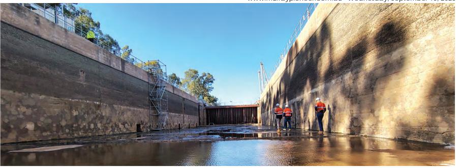
Refurbishment works on Lock 3 have finalised. decreasing the lockage process for boats by 50 per cent, with it now taking around 15 minutes to pass-through the site compared to the previous 30-minute timeframe. PHOTO: Sebastian Calderon
