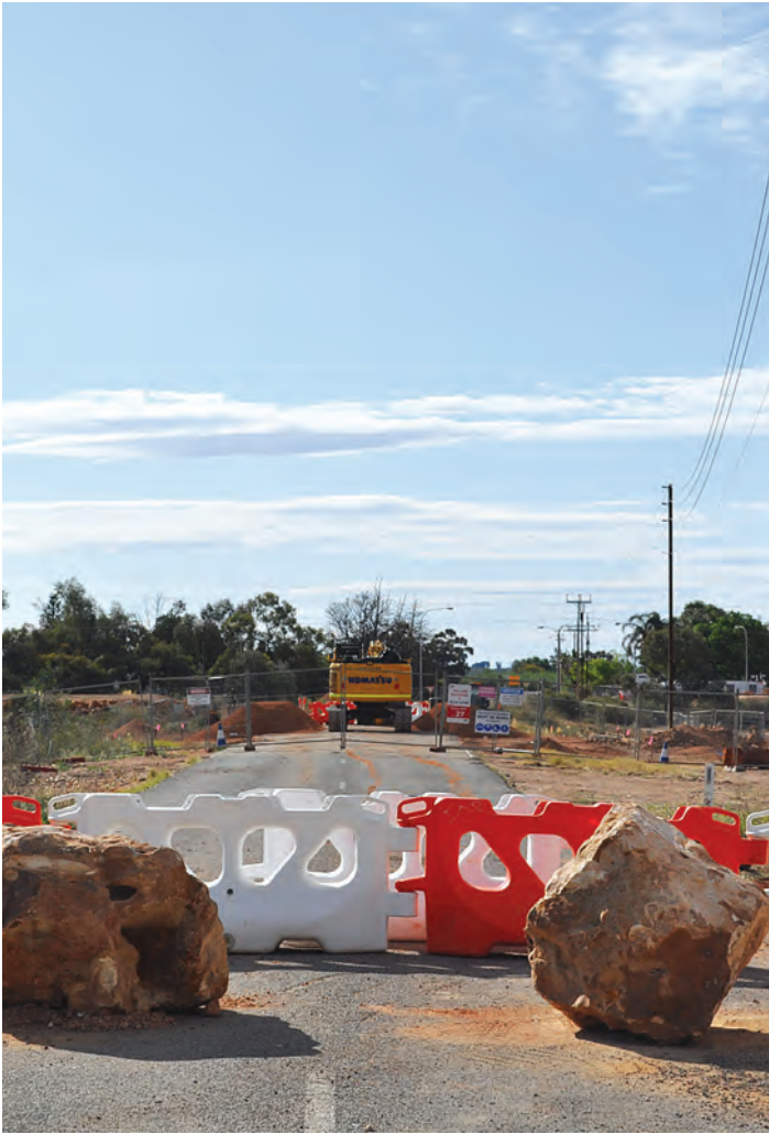
Construction works on the replacement Twentyfirst Street bridge are underway. PHOTO: Sebastian Calderon
