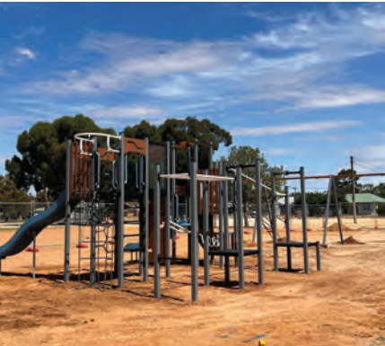
PLAYGROUND TAKES SHAPE: Works are progressing to construct the new playground at the Loxton Oval. PHOTO: supplied
