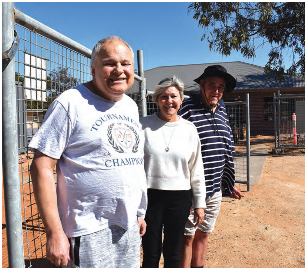
Inspecting the building site of the new share homes at Orana, Loxton, was service manager Karen Millington with residents Allen Zanetic and Trevor Lloyde. PHOTO: Stephanie Thompson
