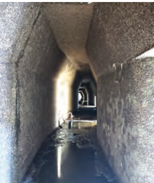
The lock 3 water chambers are essential to allow water flow, using gravity. PHOTOS: Sebastian Calderon
