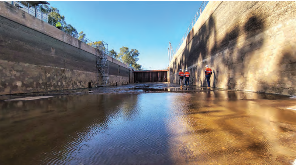
Completed in 1925, Lock 3 is drained and assessed every decade to ensure its efficiency and longevity, with current repairs taking between 14 to 16 weeks.
