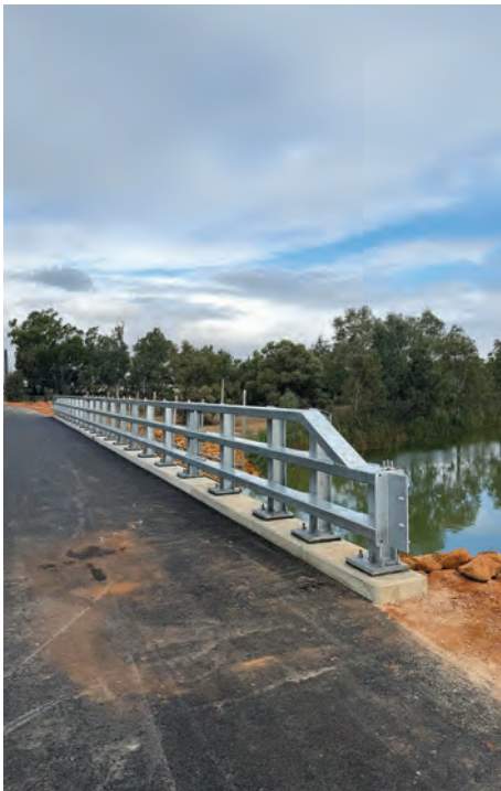
FINISHING TOUCHES: Guardrails have now been installed at the new Twentyfirst Street bridge, in Renmark, and preparations for line marking are underway. A post on the Renmark Paringa Facebook page advised an unveiling of the new bridge is “very close”, and for community members to “adhere to the safety barriers in place and wait until the road is officially opened to take a closer look”. PHOTOS: supplied
