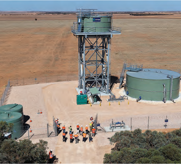
The newly built Taplan water tanks can store up to 690,000L of water, increasing storage capacity and improving the ability to provide water to the community during times of peak demand
