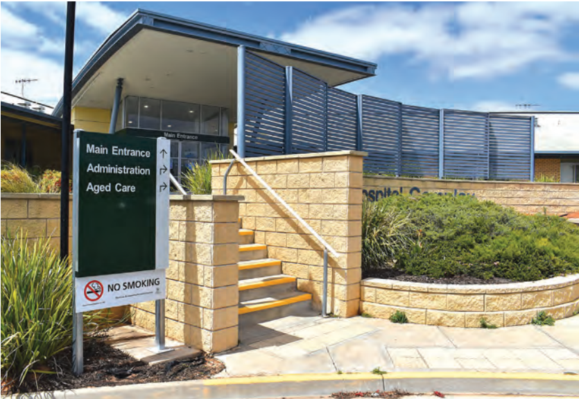
The Loxton Hospital Complex's helipad will be upgraded through a state government investment. PHOTO: Stephanie Thompson
