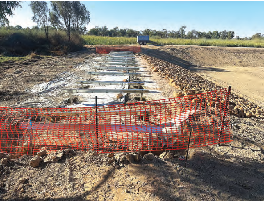
HART WORKS ROLL ALONG: Landscaping works for the Hart Lagoon Wetland redevelopment were started last week by Loxton Waikerie council. Final touches for earthworks are expected to be complete this week, with a clay liner also installed for the water storage pond. PHOTO: supplied
