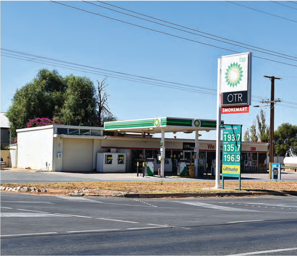
The Loxton OTR French Road store will remain open while the roundabout store receives upgrades. In July, the French Road store will close for works and is expected to reopen in December.
