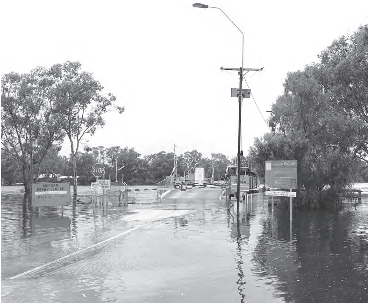
Ongoing recovery works from the River Murray flood event have delayed other Mid Murray Council capital works programs. FILE PHOTO
