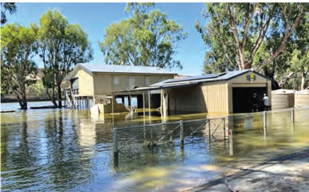
Numerous blanchetown properties were affected by the most recent flood. FILE PHOTO
