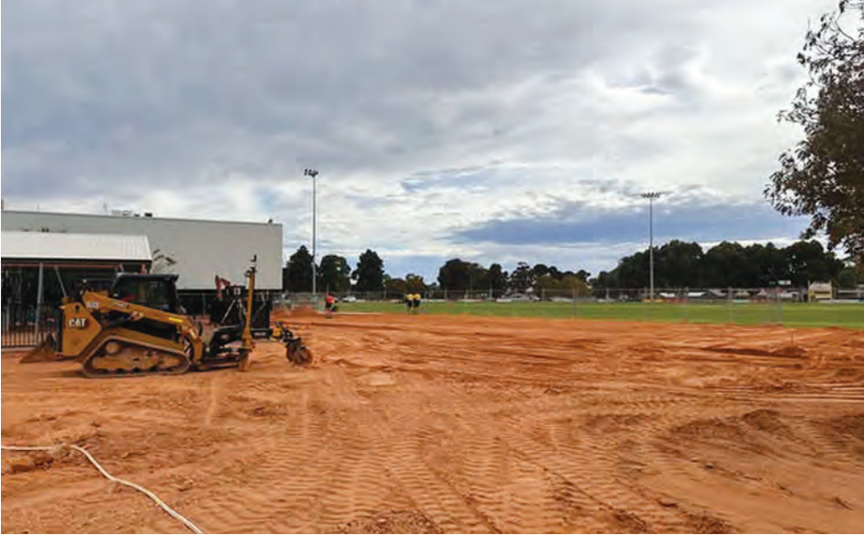
Machinery is on-site levelling the ground and preparing the surface for what it will be the new viewing pavilion.
