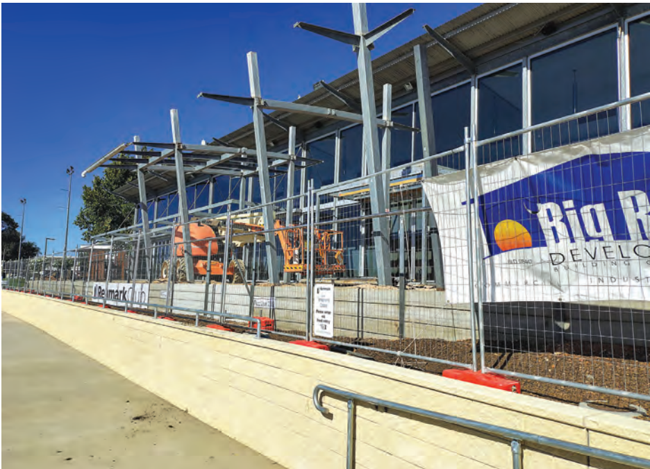
DECK TAKING SHAPE: Works have commenced on the Renmark Club’s deck redevelopment. PHOTO: Sebastian Calderon
