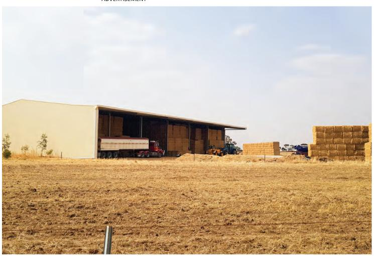
PROTECTION: A 48m x 24m x 7.5m Action Steel hay shed with a 6-metre canopy for extra weather protection. View more projects like this at the website (www.actionsteel.com.au).
