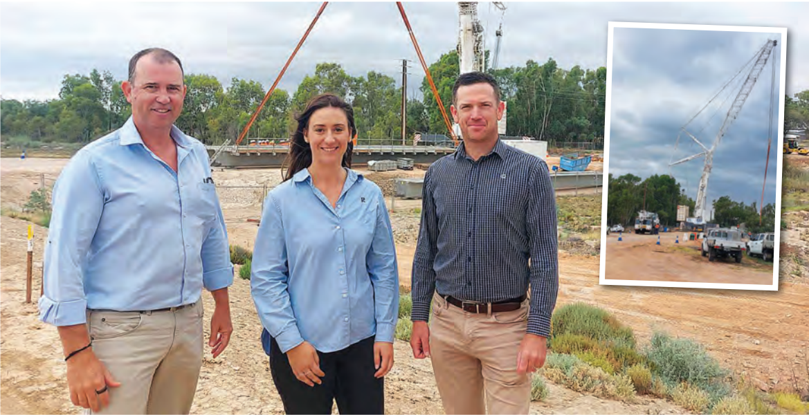
Renmark Paringa chief executive officer Tony Siviour, manager infrastructure services Shannon Baxter, and director infrastructure and environmental services Tarik Wolf, examining the construction of the new Twentyfirst Street bridge, in Renmark, last week. INSET: A 500 tonne-capacity crane was brought to Renmark to undertake installation of concrete girders for the new bridge. PHOTOS: Hugh Schuitemaker
