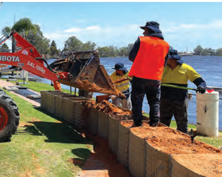
Renmark Paringa Council’s flood preparedness works included the installation of DefenCell sandbags along the Renmark riverfront. PHOTO: supplied
