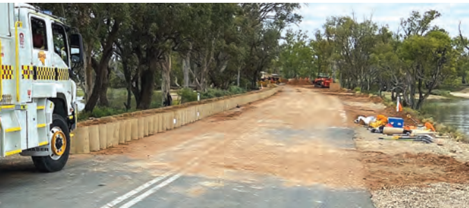
A temporary earthen levee and DefenCell sandbags have been deployed on the west of Lake Bonney. PHOTO: Facebook
