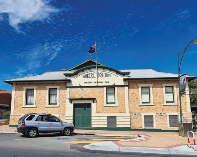
A petition outlining concerns about the state of the Waikerie Institute/ Soldiers Memorial Hall is being circulated around Waikerie. PHOTO: Christine Webster
