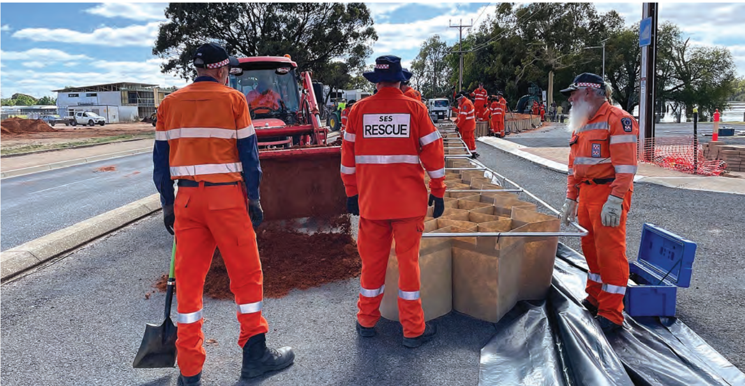
Works have continued on the installation of a DefenCell barrier along the Berri riverfront, with council also mobilising to protect other sections of Riverview Drive. PHOTO: Facebook
