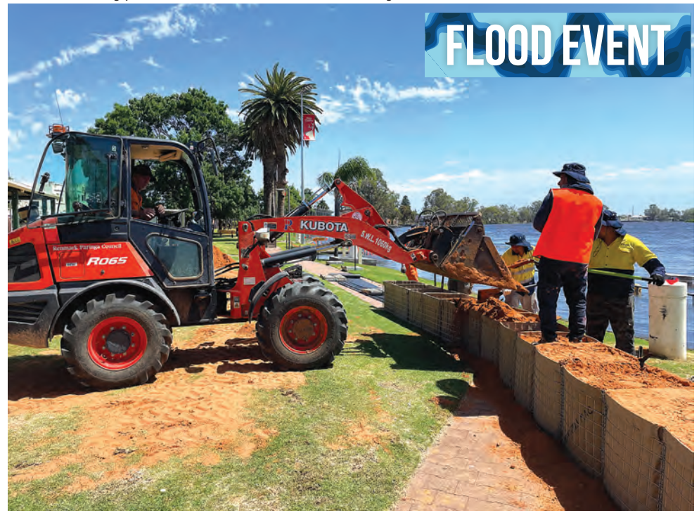
Renmark Paringa Council staff, SES volunteers and Costa Group workers constructing the DefenCell sandbag barrier at the Renmark riverfront last Wednesday. PHOTO: supplied
