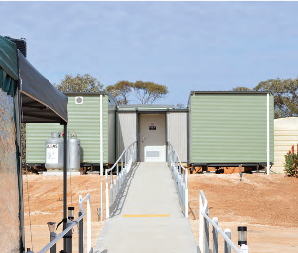
New male/female toilets and showers at the camp, with disabled toilets and ramps.
