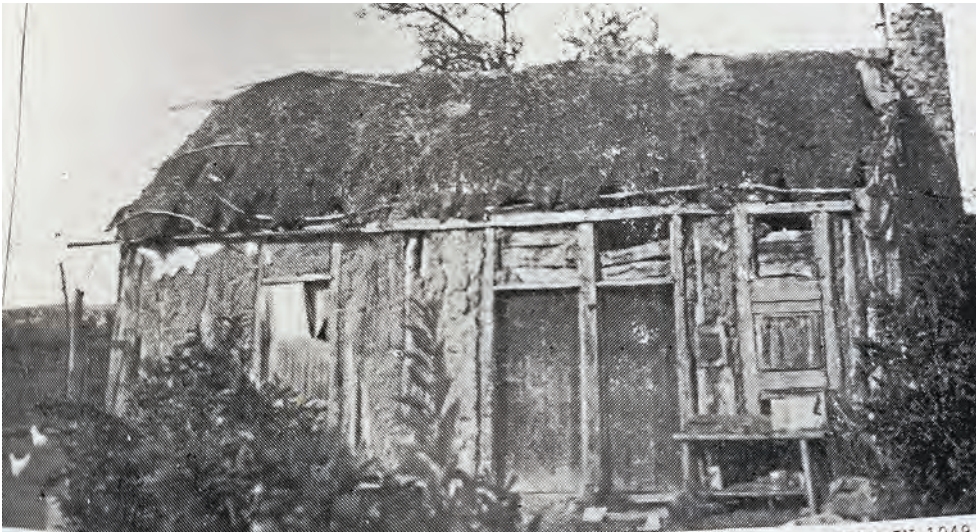
The first Lutheran Church the small Bookpurnong congregation had for worship was built of pine slabs, plastered with a mixture of swamp clay and sand and covered with a thatched roof, situated further down past the current Church on Schwarz Road, Bookpurnong. PHOTOS: supplied
