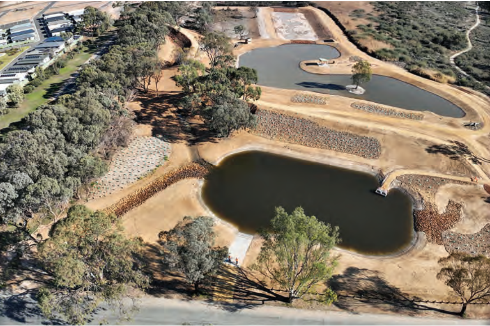
A Hart Lagoon Wetland overview. PHOTOS: supplied
