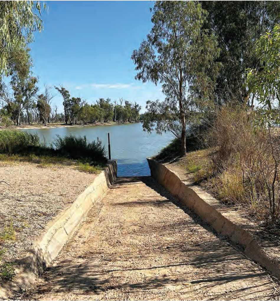
Renmark Paringa Council last week began upgrades on the Lock 6 Boat Ramp. PHOTO: supplied
