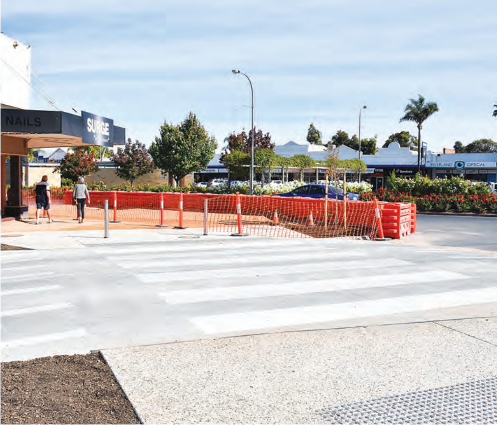
Renmark Paringa Council last week commenced stage two works for the raised pedestrian crossing at the 180 Murray Avenue. PHOTO: Alexandra Bull
