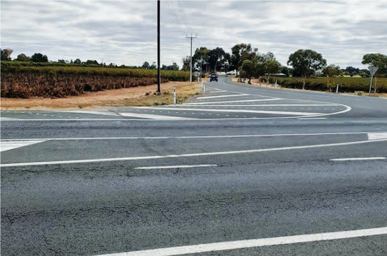
An example of a turn-off a Loxton district man says has effectively been narrowed by the installation of audio tactile line marking. PHOTO: supplied
