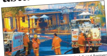
CFS crews from Waikerie, Blanchetown, Cadell and Barmera worked tirelessly for two hours to control the blaze at the Waikerie Hotel Motel on Sunday morning. PHOTO: Maddie Miller
