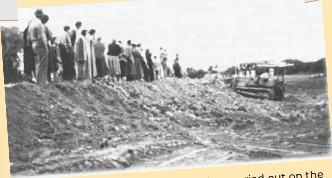
Curious locals watching work being carried out on the flood bank in Cobdogla.
